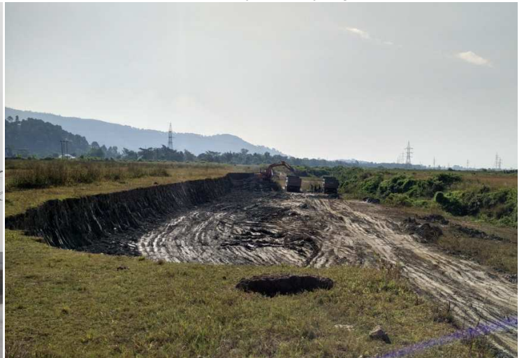
Development of Waterbody at Mayang Langjing, Imphal West
